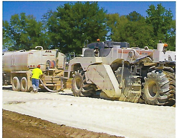
Soil stabilization in process
